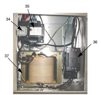
FIG. 5: Transformer Compartment Electrical Components
